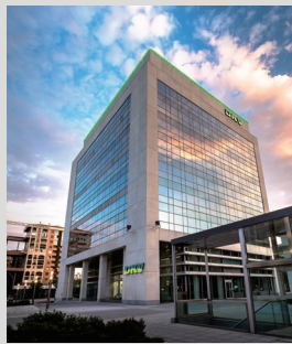
HQ Mansion of DKV, Spain
